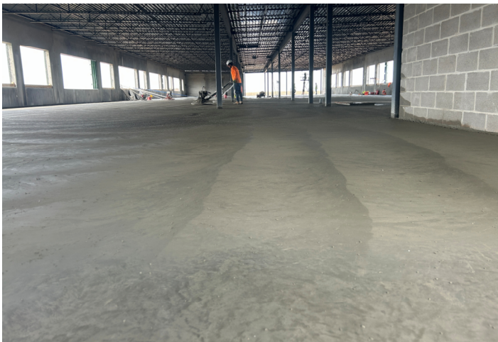
Pouring & Finishing Classroom Area Slab on Grade & Metal Deck
