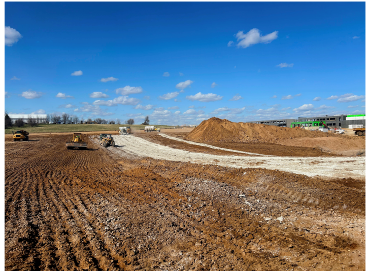
Grading (Lime Stabilization) by the Baseball Field
