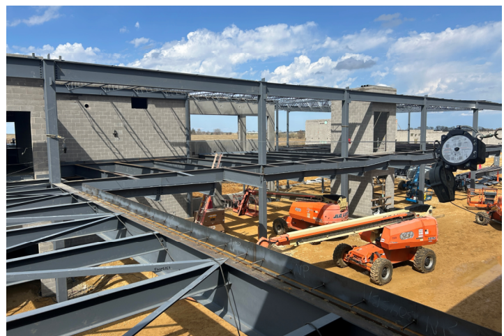
Setting Clerestory Steel Beams, Joist & Decking
